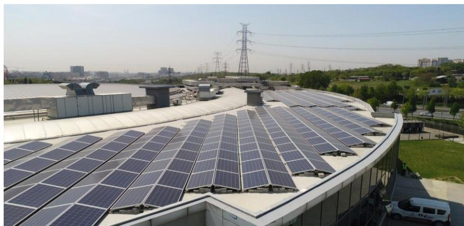
**Figure 17.** East–west orientation application view 2.
