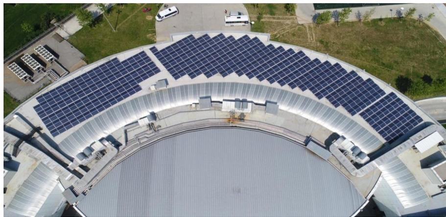
**Figure 16.** East–west orientation application view 1.
